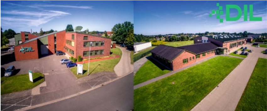
DIL Institute site – 9.000 square metres working space.
